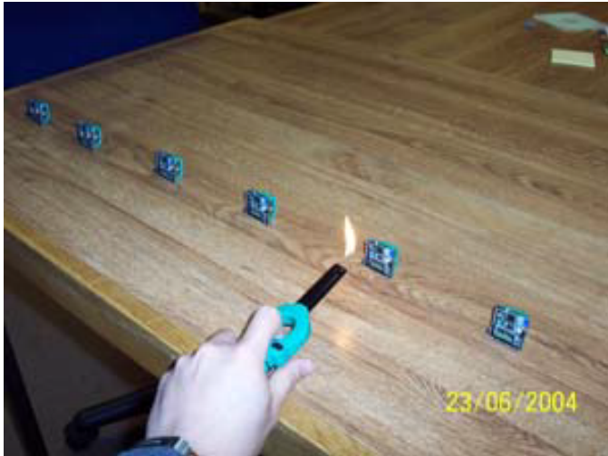
Fig. 4. Demonstrating a distributed intelligent wireless fire alarm system
